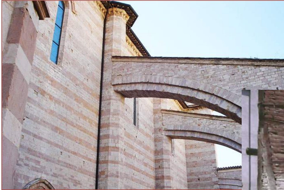
Flying buttresses Assisi, Central Italy
